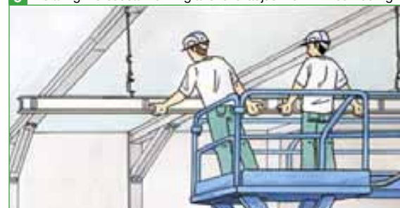
3 Installing the busbar trunking and level adjustment without tooling
